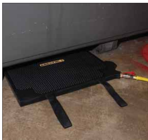
◀ Preparing to lift a CNC machining center.
